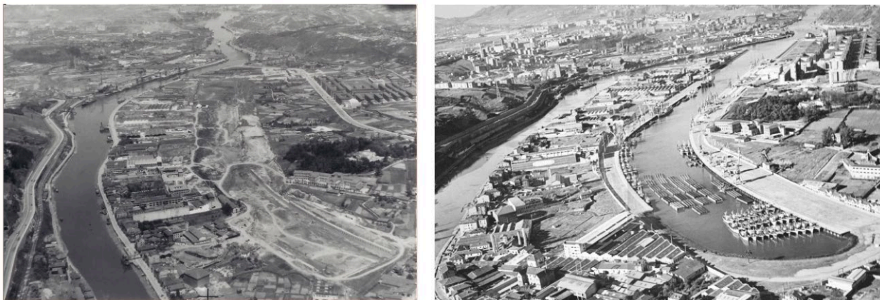
Figure 15 - Zorrotzaurre in 1959 Right photo: Zorrotzaurre in 1970 after the open of Deusto Canal
