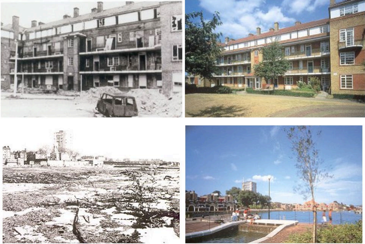
Figure 8 – Photos from before and after LDDC actions - Top Left and Right: Before and After Acorn Walk, Surrey Docks - Bottom Left and Right: Before and After Shadwell Basin (Source: Monograph Archive of The LDDC History Pages, 1981-1998)
